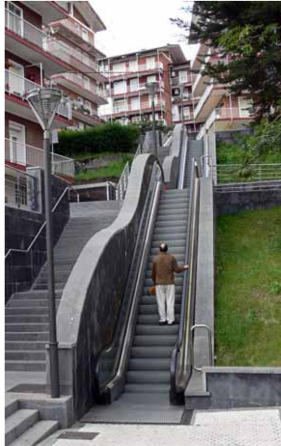
**Outdoor escalators** are relatively recent systems compared to indoor ones which were first installed at the end of the 19th century. Technological innovation in this field has led to the manufacture of system components that can be exposed to the weather with sufficient reliability to ensure uninterrupted service.
